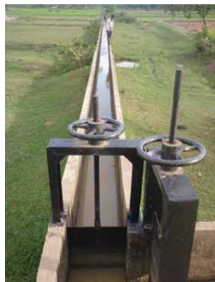
Concrete canals at O Krasar, Kep province
